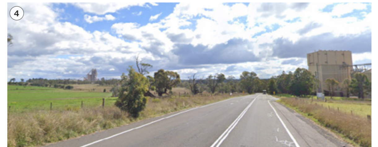
View from Berrima Road looking west - the Ingham Mill can be seen in the middle-ground and the Boral Concrete Works silos in the background
