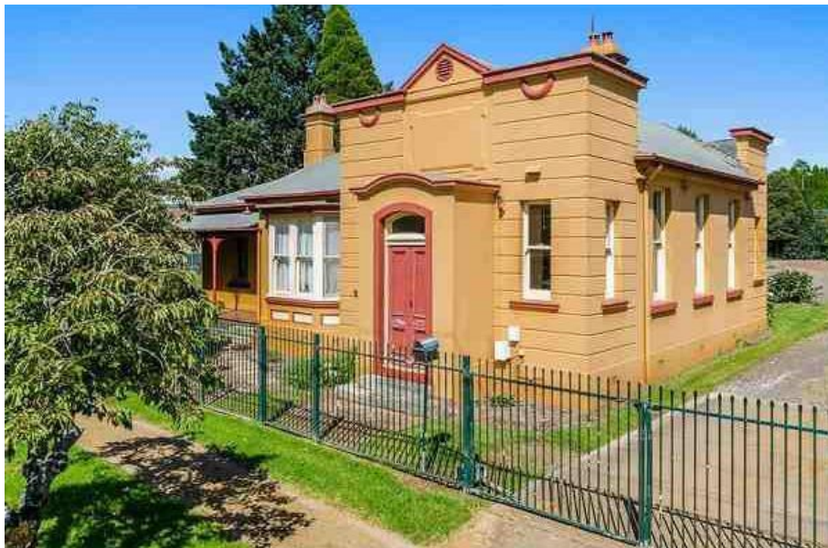
Above: Photo of exterior of bank in 2018 with previous, more sympathetic colour scheme (Source: https://www.realestate.com.au/property/67-69-hoddle-st-robertson-nsw-2577 , accessed 2021).
