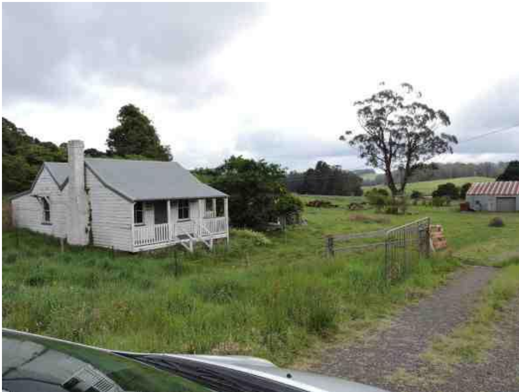
Above: 'Redbank Cottage' from the Illawarra Highway (2020).
