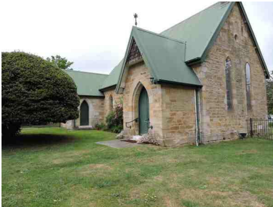
Above: Photograph of the northern side of St John's Church showing the entry vestibule (2020)
