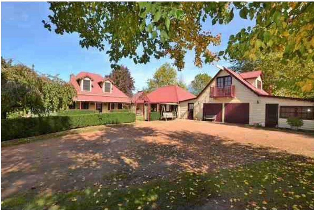
Above: Twin Creeks buildings 2015 (Source: https://www.realestate.com.au/property/140-old-kangaloon-rd-robertson-nsw-2577 )
