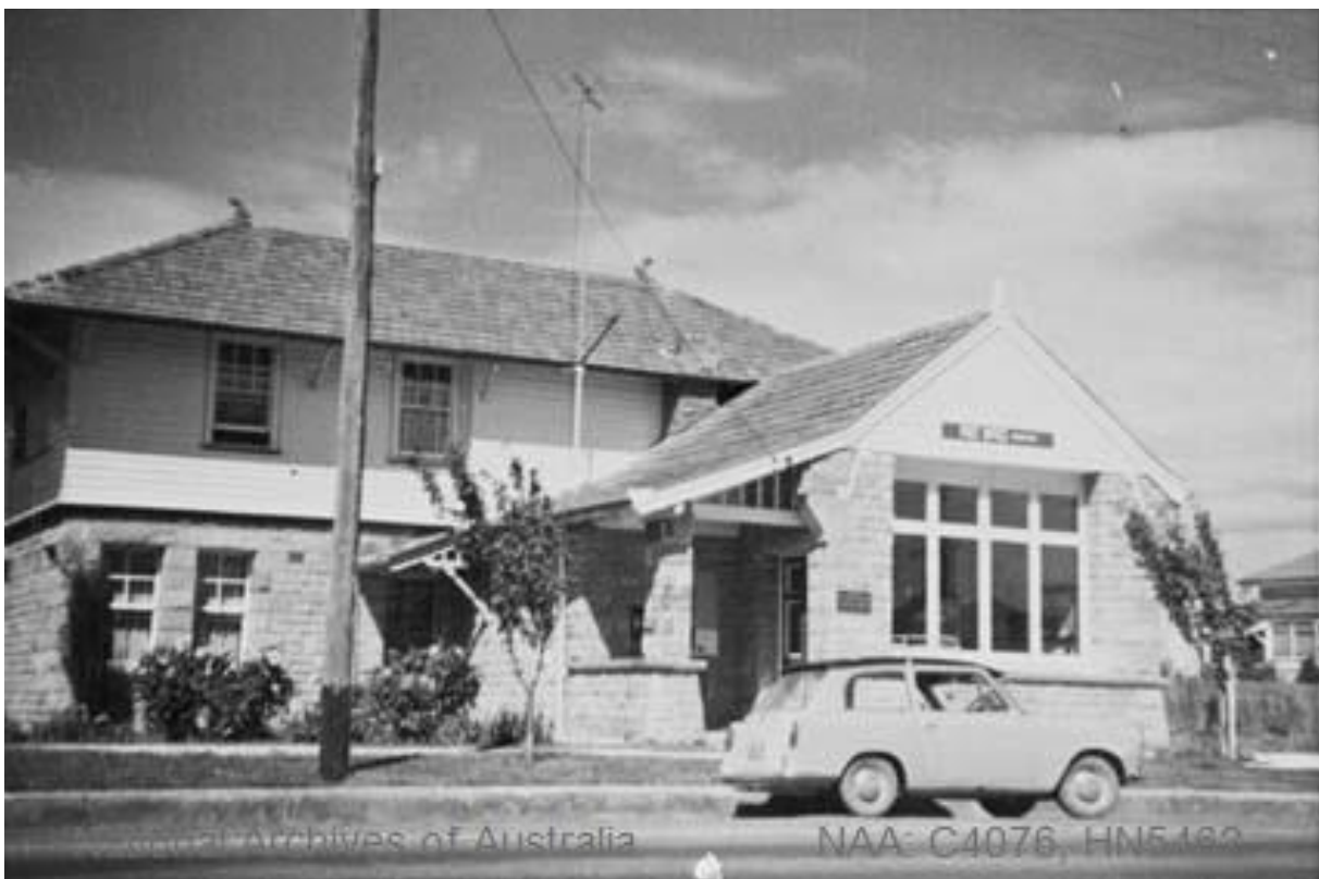
Above: 1969 image from National Archives of Australia shows that following the 1961 earthquake the chimney has been removed down to roof level and that the front wall of the public area has been rebuilt with a new squared window with timber infill above. The elegant turned timber support columns to the street were replaced by a stone pillar possibly from the demolished wall and/or demolished chimney. The building continued to be used as a post office until 1994 (Source: National
