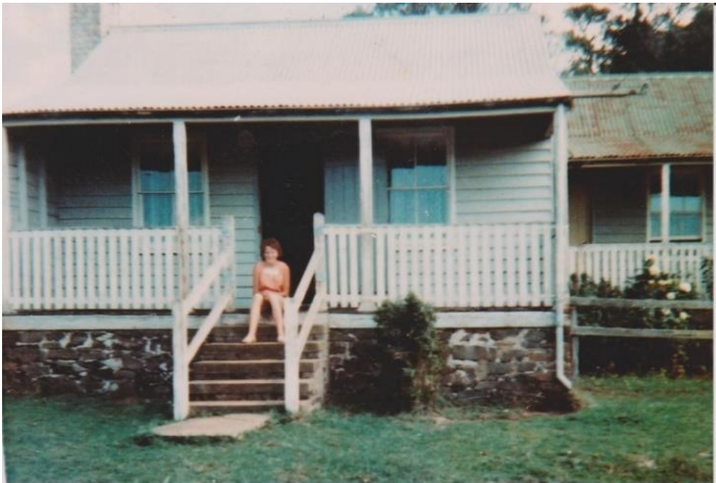
Above: “Jeff Fisk’s old house near Butter Factory occupied by the Handley Family until 1973”. This image shows the earlier 6+6 pane window section to right and the 2+2 pane window in the later added section to the left (Source: Robertson History Group, obtained 2022).
