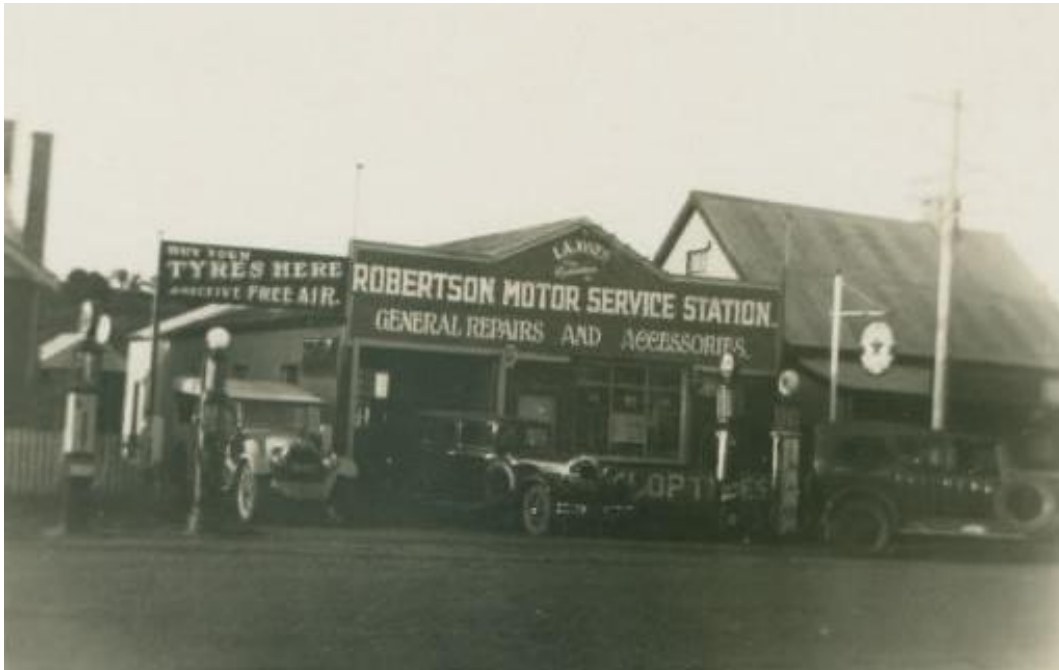
Above: image from the early 1930s showing Lenville Jones' service station at centre and the pitched gable roof of 28 Hoddle Street at right. Side window can be seen in the upper floor of No. 28 and at that time it featured a straight verandah and no parapet. (Source: Robertson History Group)
