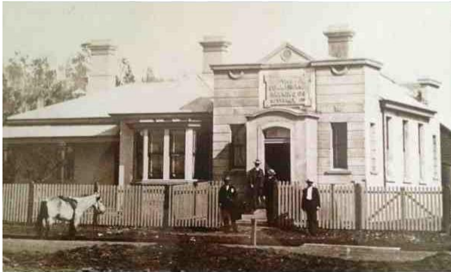
Above: Historical photograph of the CBC Bank c.1900 (Source: https://www.realestate.com.au/property/67-69-hoddle-st-robertson-nsw-2577 ).
