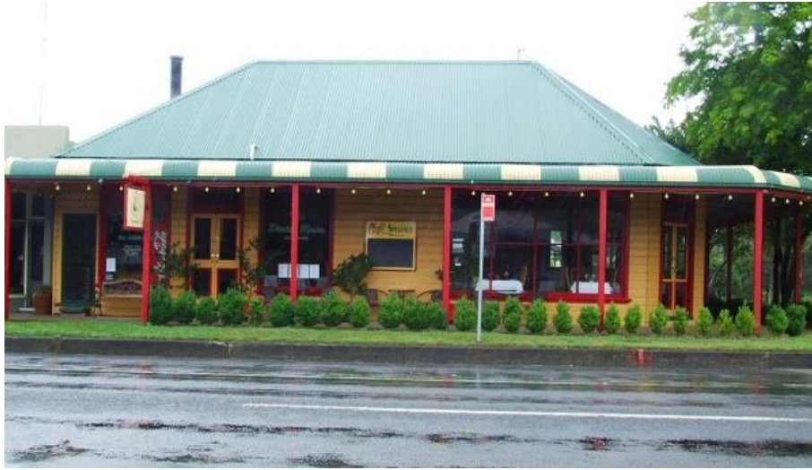
Above: image of 42 Hoddle Street, Robertson showing the previous green roof and verandah striping. (Source: https://mapio.net/s/83600667/ .)
