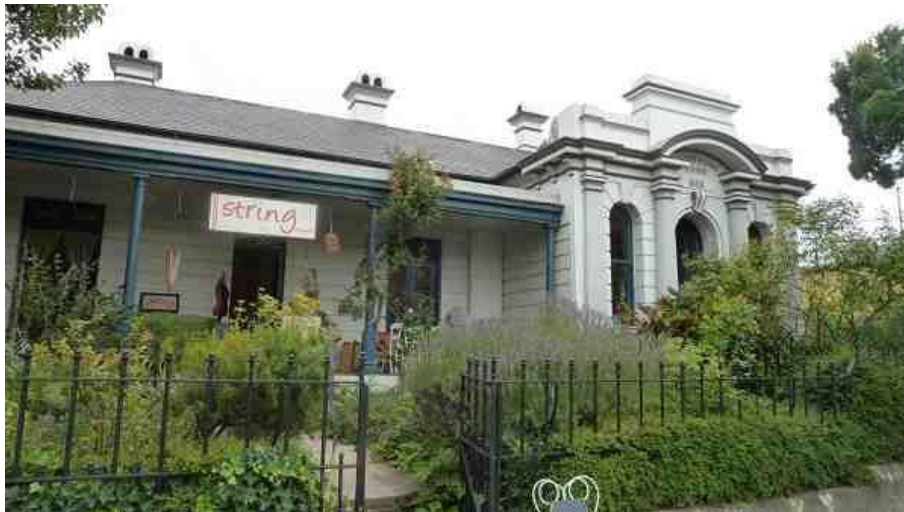
Above: Former CBC Bank at Braidwood, NSW (Source: CBC Officers Club Inc website http://www.cbcbank.com.au/images/Branches/NSW/NSW%20Country/NSW%20Country%20A-B/Braidwood/Braidwood%20from%20st%20JN%20P1020878.JPG ).
