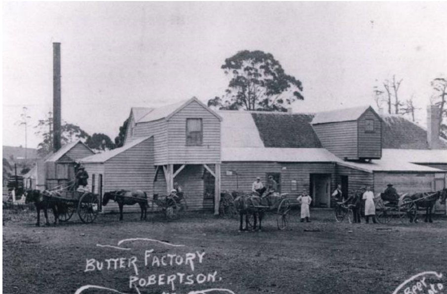
Above: Undated image of the 1889 Robertson Butter Factory from BDHS collection via the Southern Highland News. Note the upper floors in this image are now missing.
