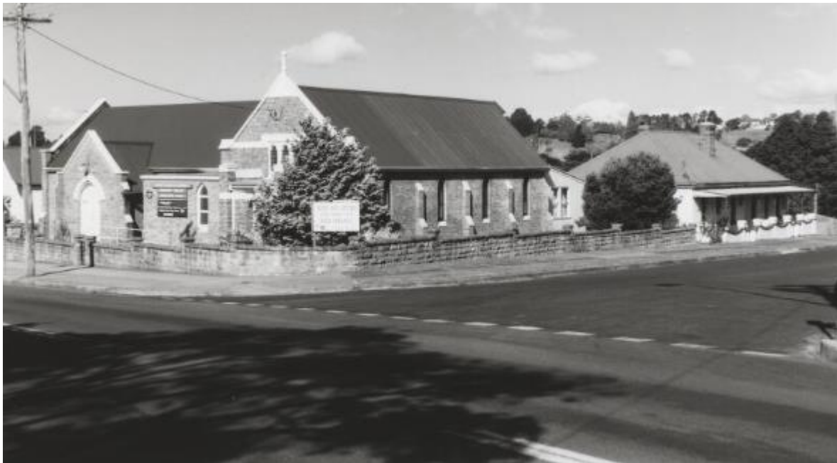
Above: Image from 1996 of Uniting Church Moss Vale, Spring and Argyle Streets [picture] Creator: Deane, Robert, 1937- . https://nla.gov.au/nla.obj-143052353/view
