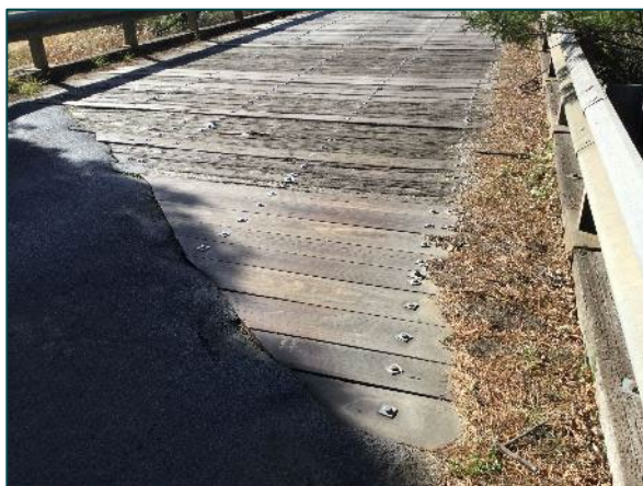
Plate 24: Timber decking, facing east.
