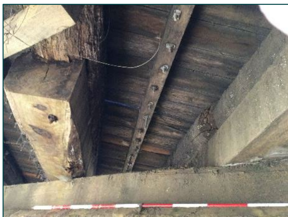
Plate 22: Detail of timber work and reinforcing atop the pier, facing east.
