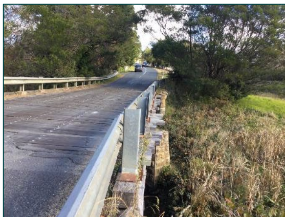
Plate 25: General view of bridge showing decking and railing, facing west.
