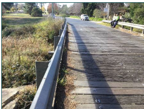
Plate 26: Bridge decking and railing facing east towards Fitzroy Inn.
