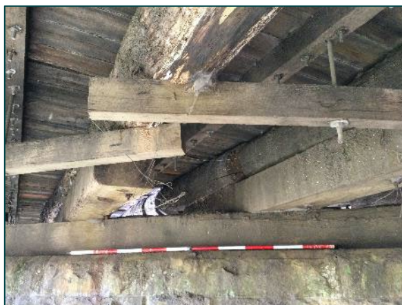
Plate 23: Detail of timber work and reinforcing atop the pier, facing east.
