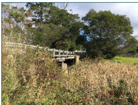
Plate 27: Overview of northern side of bridge facing southwest.
