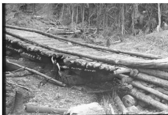
Plate 2: Man standing beneath Corduroy Bridge (log bridge) c.1886 (source: Trove, n.d.)
