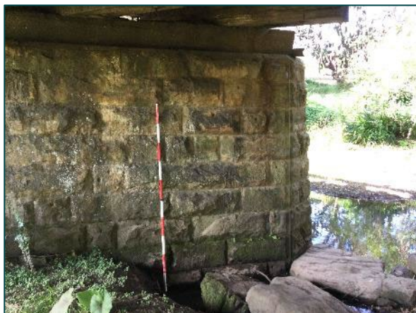
Plate 18: West face of central pier facing east.
