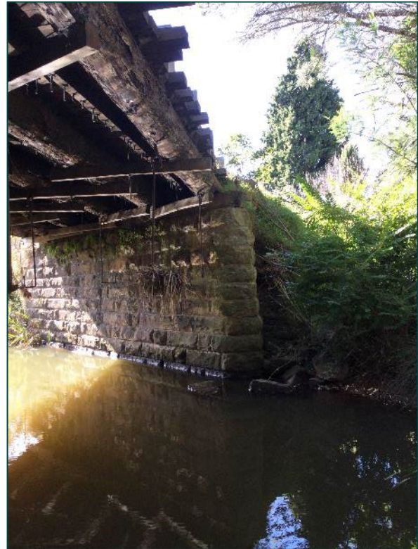
Plate 13: underside of eastern span and eastern abutment, facing east
