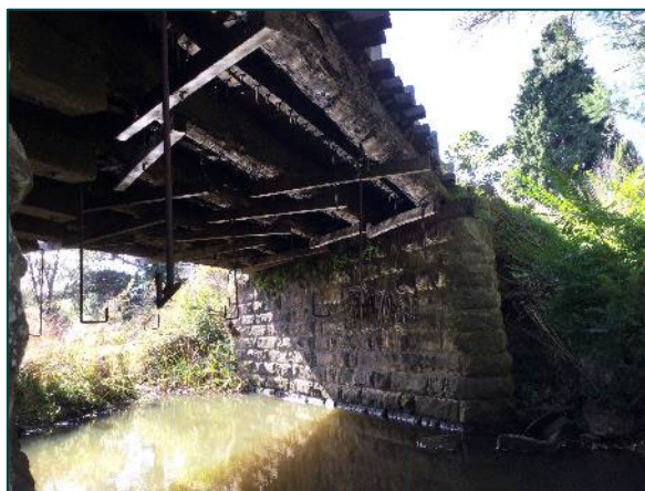
Plate 21: Underside of eastern span showing timber work, facing east.
