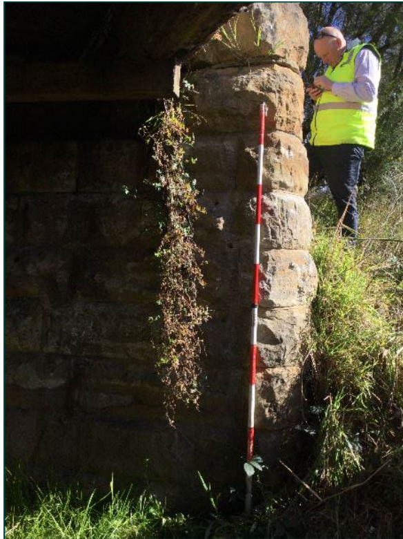
Plate 12: northern side of western abutment, facing west
