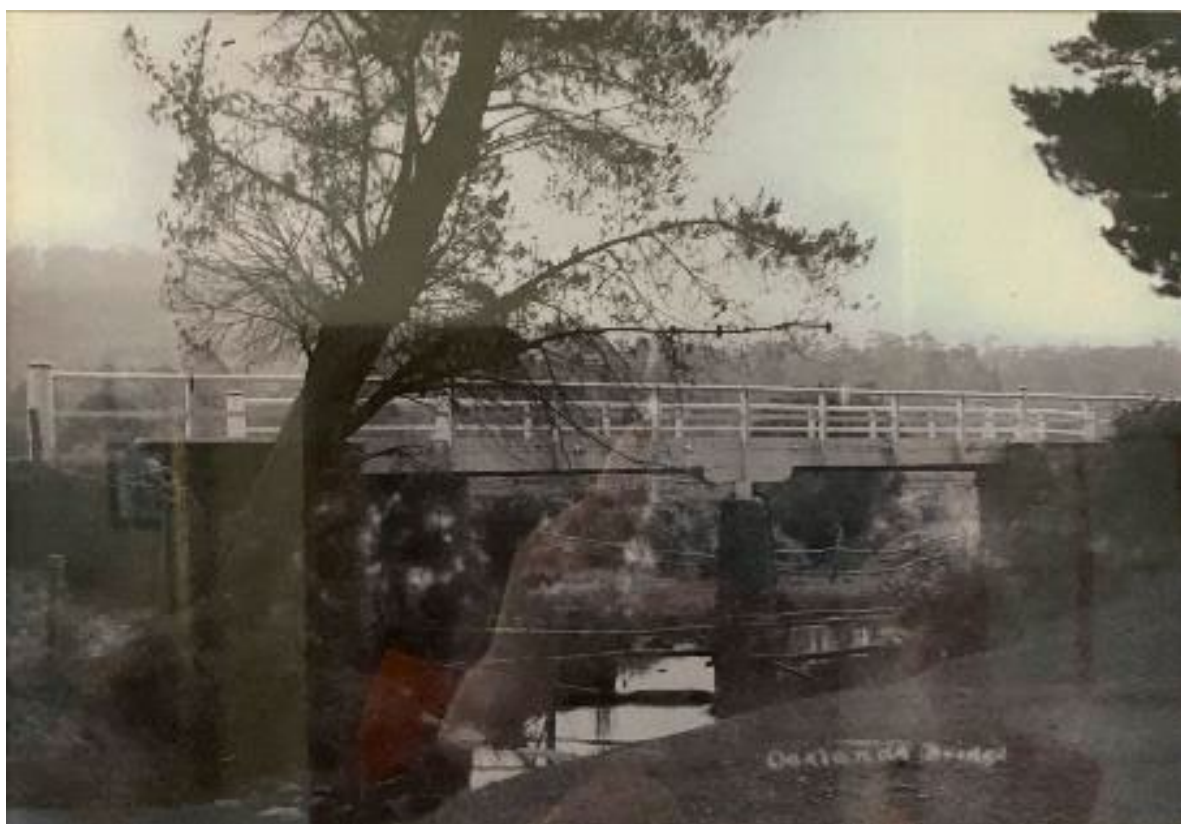
Plate 11: Oaklands Bridge (Nattai Creek Bridge) (Fitzroy Inn 2023, N.D.)
